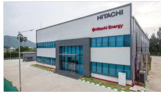
New valve and C&P 1 factory: Chennai, India
