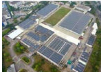
Photovoltaic system (Dong Guan Keihin)
