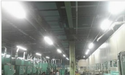
Replace with LED (Tomi Plant)
