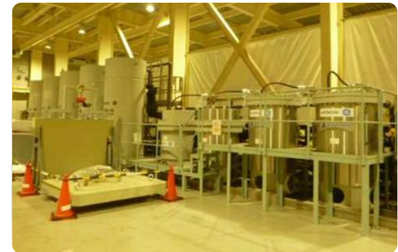
Subdrain and other cleaning facilities *1
