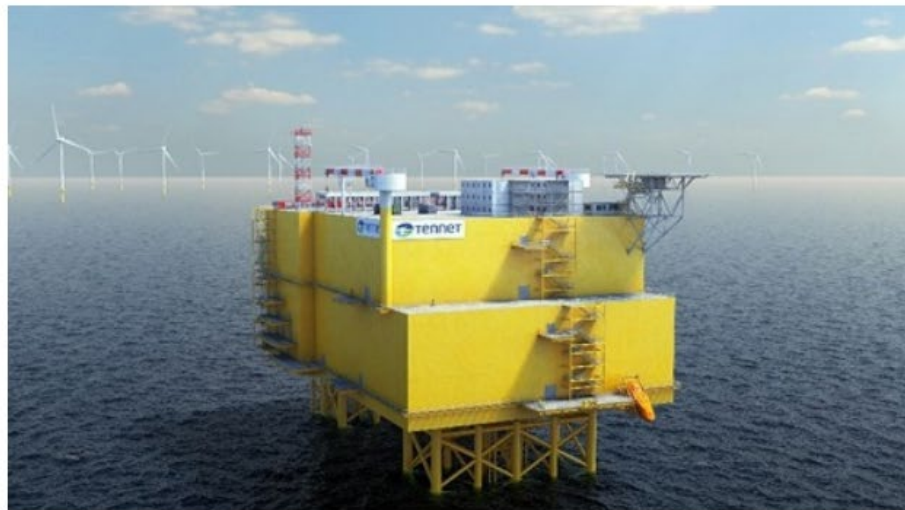
2GW offshore platform. Photo courtesy of TenneT
