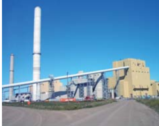
Keephills 3 power plant (Canada)
