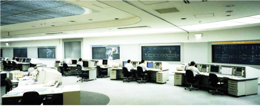
Fig. 7—Central Command Center of Teito Rapid Transit Authority. Teito Rapid Transit Authority is moving its integrated traffic management system away from surveillance of all lines via monitors and toward providing functions such as control information services and cooperative control among lines.
