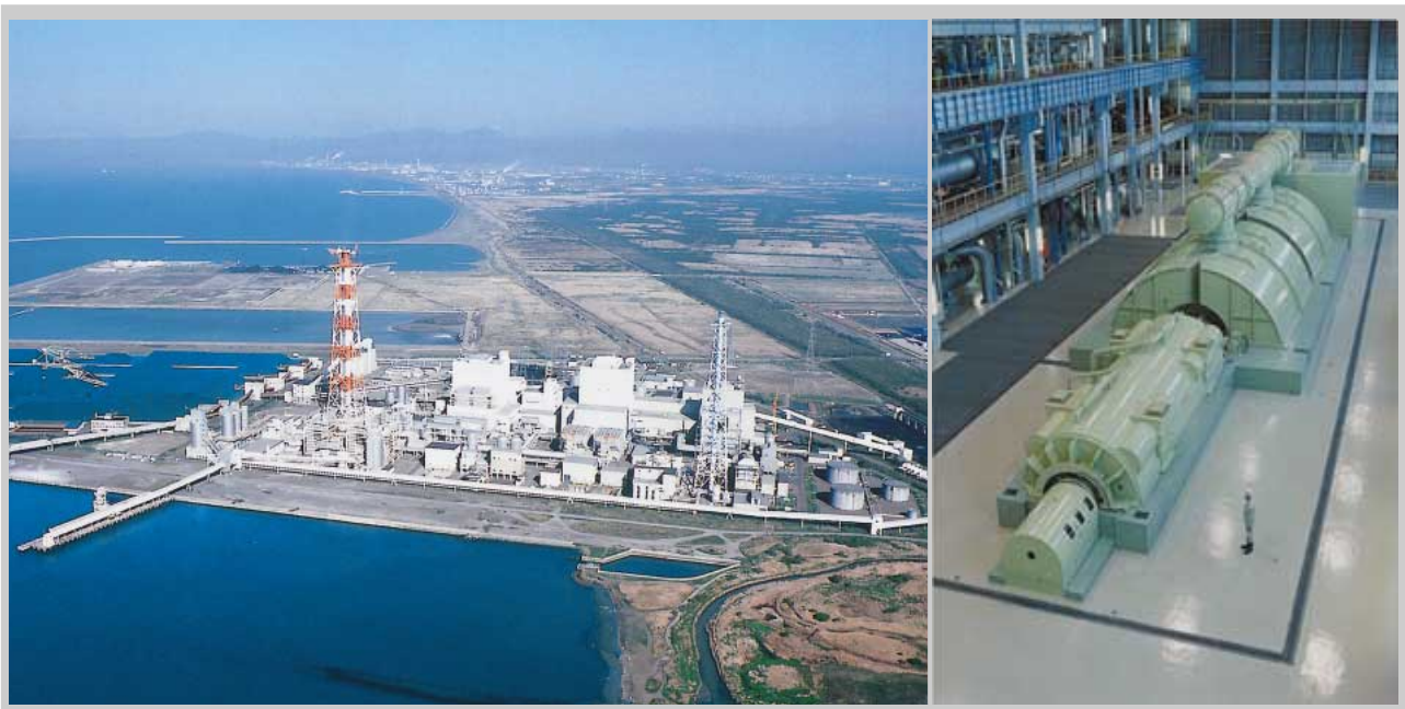
Fig. 1—Bird's-eye View of the Completed of Tomatoh-Atsuma Power Station of Hokkaido Electric Power Co., Inc. (left), and the 700-MW Turbine Generator for the No. 4 Unit (right). The Tomatoh-Atsuma Power Station is located between the towns of Tomatoh and Atsuma, and with the completion of Unit No. 4, has an output capacity of 1,735 MW, making it the largest power station in Hokkaido.
