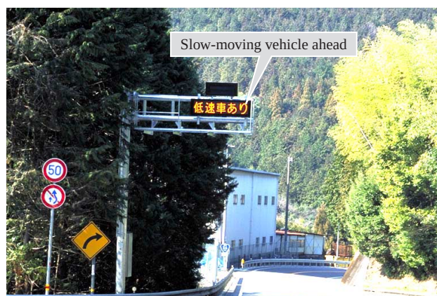
Fig. 5—Information Displayed on Variable Message Sign. Warnings are displayed in text format on the message sign to draw drivers' attention to conditions ahead of curves in the road.
