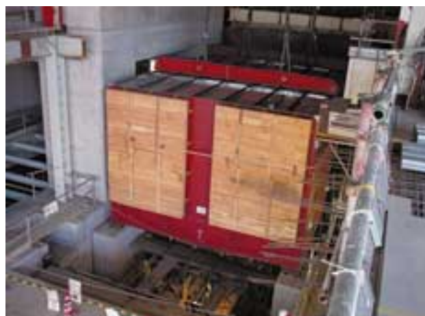
Fig. 6—Condenser Installation. The condenser was brought in by a special dolly from the boiler side in the turbine building and installed underneath the turbine generator frame. (Photo: lower body of the condenser)
