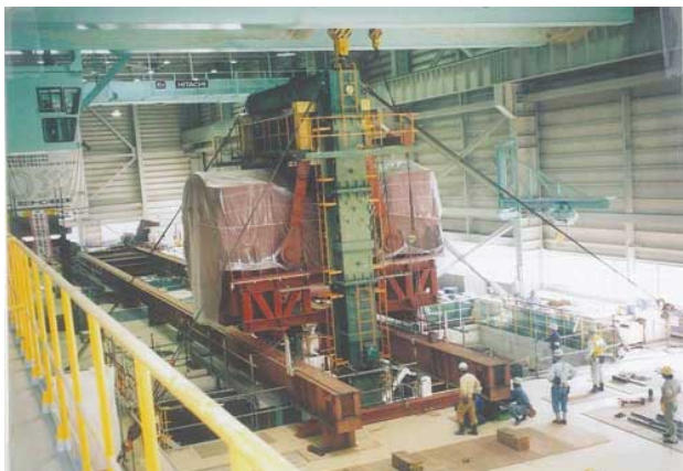
Fig. 5—Generator Installation. The jack and rails used for installing generators were shared when both generators were installed.
