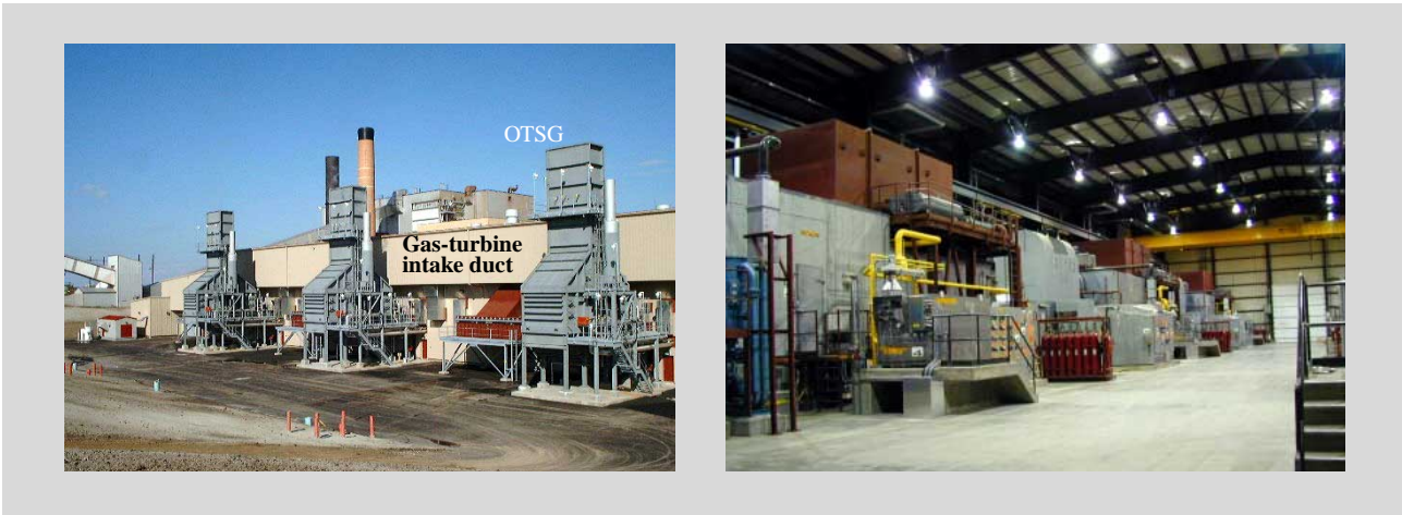
Fig. 1—Re-powering System Installed at Queen Elizabeth Power Station (on the left); H-25 Gas-turbine Units (right).
