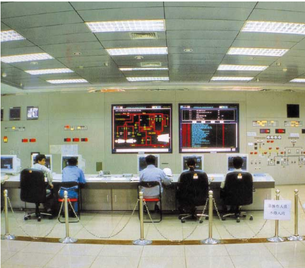
Fig. 3—Unit Control Room for Jiangxi Jiujiang Phase III Power Generating Co., Ltd.
