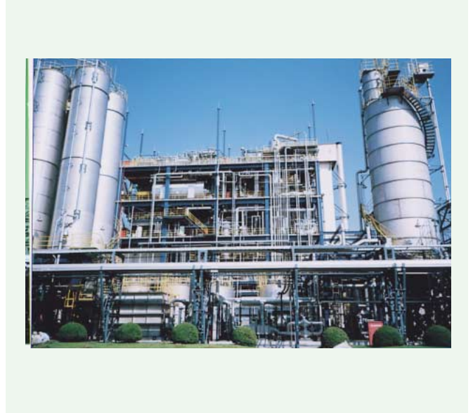
PBT continuous production plant for Mitsubishi Chemical Corp.
