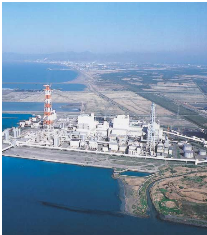
Tomatoh-Atsuma Power Station
