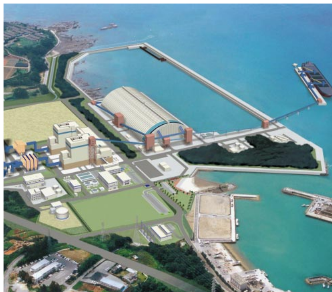
Expected Outline of Kin Thermal Power Station The site was prepared by reclaiming land from Kin Bay in addition to site preparation work where the former power plant had been situated.
