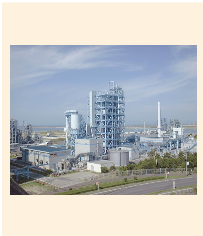
View of EAGLE pilot plant
