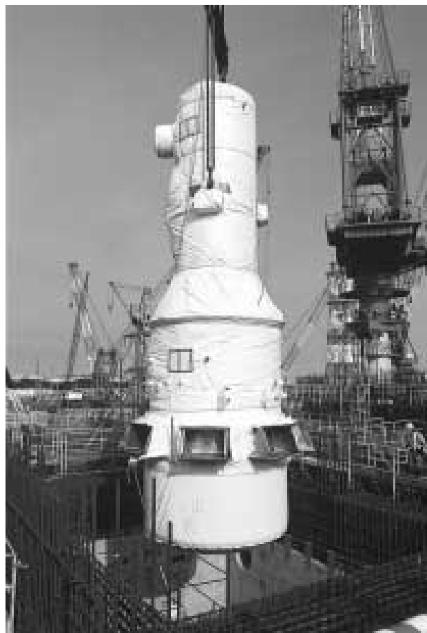
Fig. 3— Installation of Apparatus for the Concentration of High-Level Liquid Waste; Corrosion-Resistance Techniques Were Gathered on a Worldwide Scale for Application to This Waste-Reduction Vessel.
