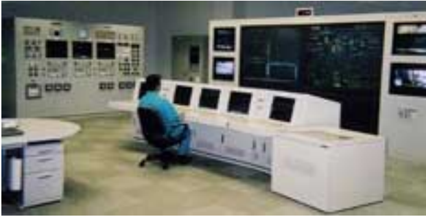
Fig. 5— Central Control Room. The central control room contains an automation panel, a large screen, and auxiliary panels for independent operation.
