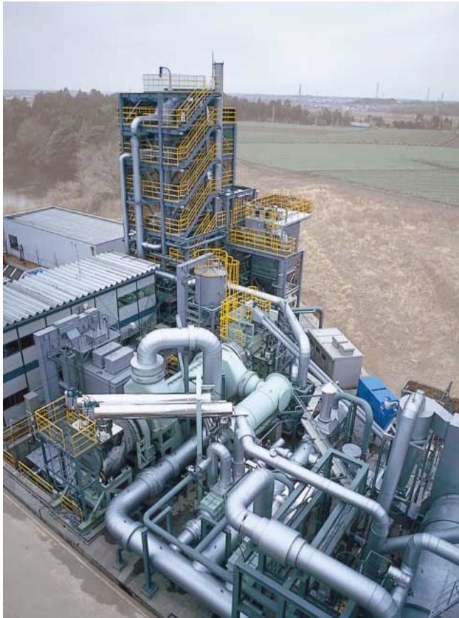
Kiln-type gasification/melting system pilot plant (Hitachinaka City, scale of process: 20 t/d)
