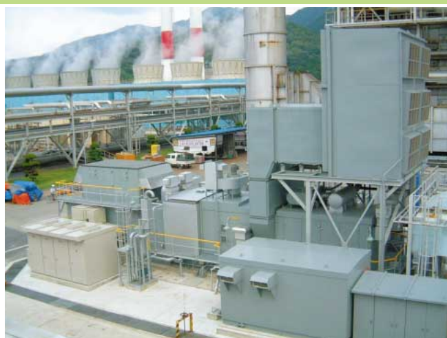
H-25 gas turbine at LGPC Yosu Plant
