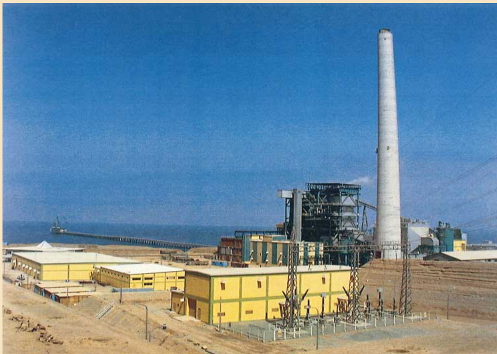
Peru, ILO No. 2 Thermal Power Plant—125-MW Coal-fired Unit No. 1
