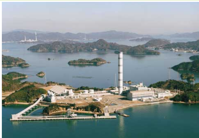
Bird's-eye view of the 250-MW PFBC power plant delivered to the Chugoku Electric's Osaki Power Station
