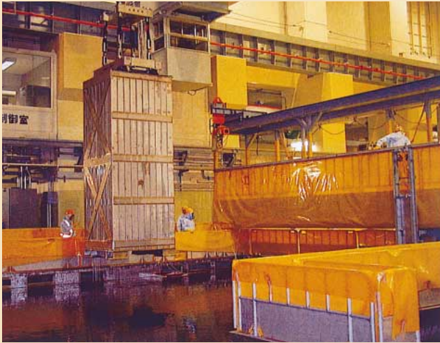
Existing stainless-steel rack detached from SFP
