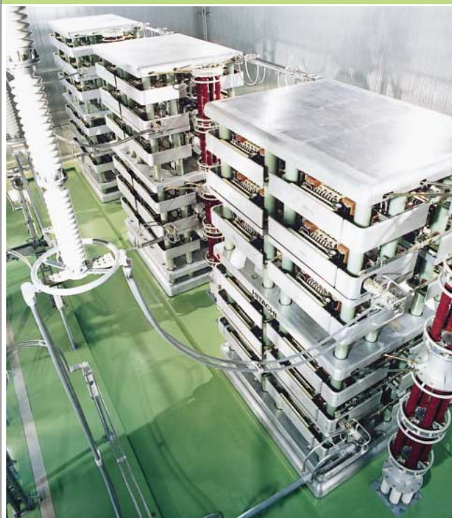
The 700-MW thyristor valve (250-kV/2,800-A quadruple-valve unit)
