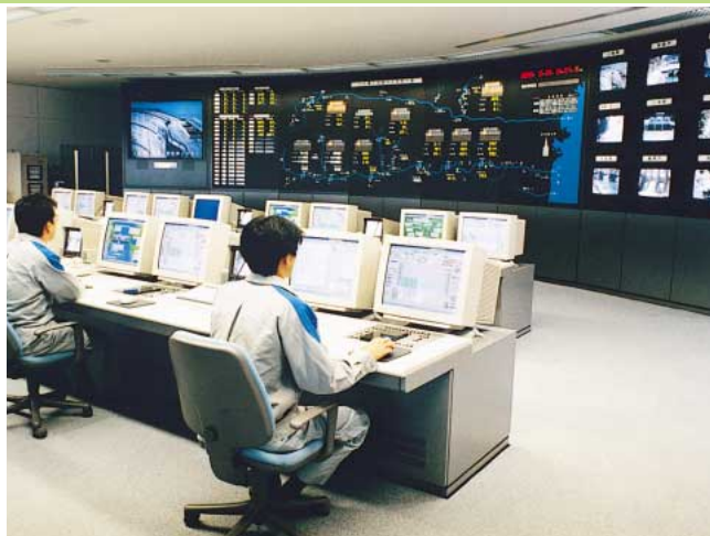
Total-dam-management system at the Hyuga Power Office of Kyushu Electric Power Co., Inc.
