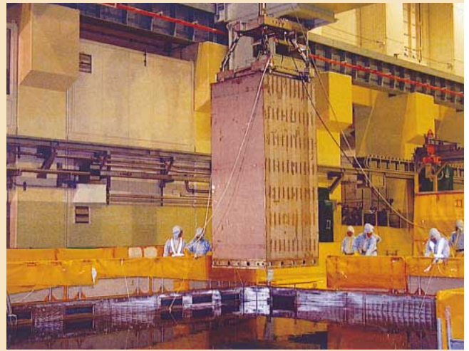
New high-density BSS rack installed in SFP
