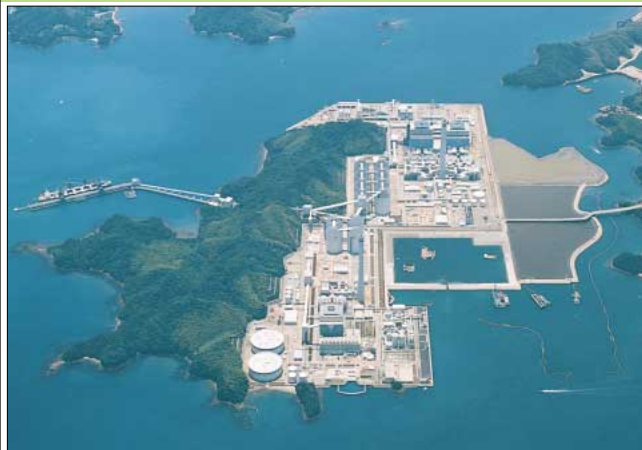
State-of-the-art coal-fired boiler facilities Top: Electric Power Development Co., Ltd. Bottom: Shikoku Electric Power Co., Inc.
