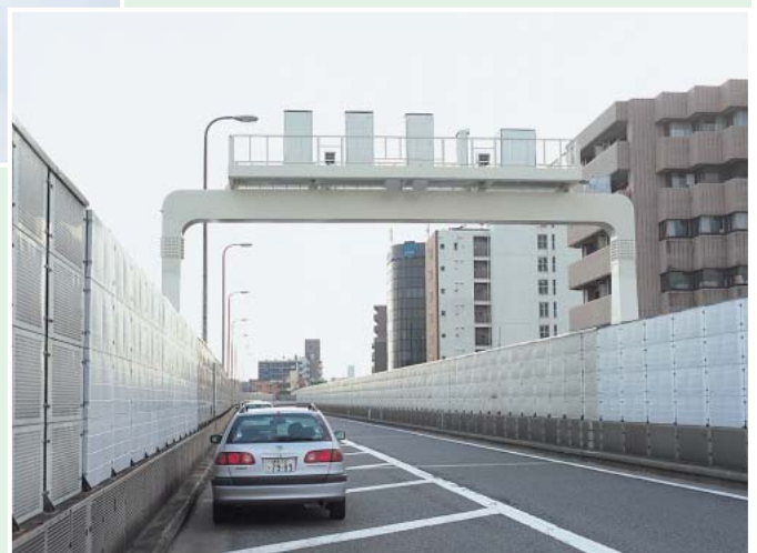
Equipment for free-flow system installed on test course (above left), and exit lane of Metropolitan Expressway in Tokyo (below right)
