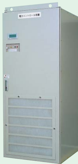
115-kW permanent magnet synchronous generator (above left) and 100-kW power conditioning system (below right)
