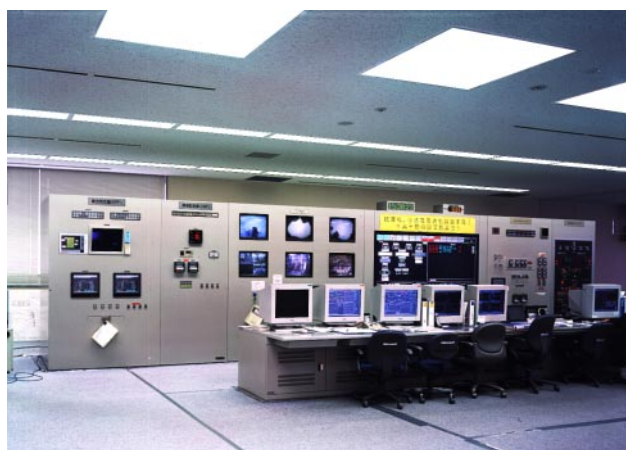
Fig. 5—View of Main Operator Control Panel and Expanded-Display Devices in Central Control Room.
