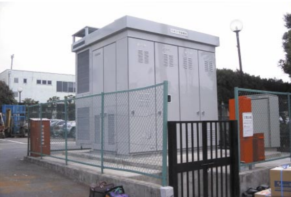
Fig. 6—External View of the 22-kV/6-kV Large-capacity Mini Substation.
