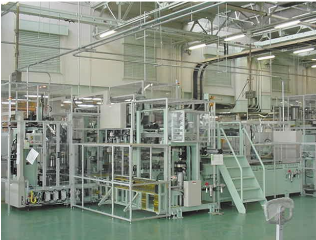
Fig. 5—Motor Winding Production Line for HEVs. Production capacity is 5,000 units per month.
