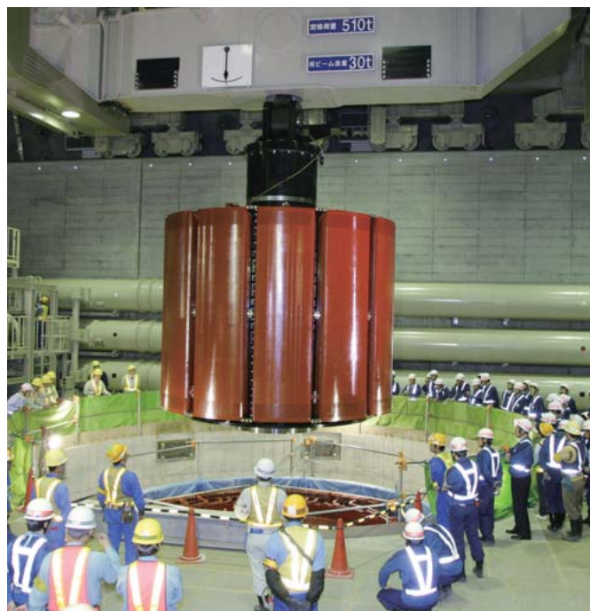
Rotor of the 525-MVA/464-MW generator-motor installed at the Kannagawa Power Station of the Tokyo Electric Power Co., Inc.
