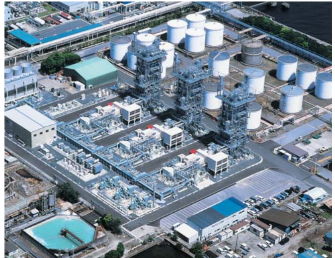
External view of the Goi Power Plant of Goi Coast Energy, Ltd.
