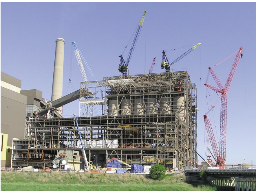
Fig. 1—Photo of Project Construction in Progress, May 2005.
