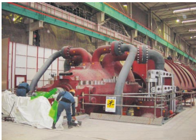
Fig. 5—Installation Status of Main Steam Lead Pipes and Reheated Steam Pipes.
