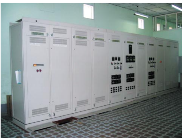
Fig. 2—External View of HIACS-MULTI 1000. By applying a turbine-control system that integrates the functions for controlling both the gas turbine and the steam turbine, it is possible to provide a compact monitoring and control system.
