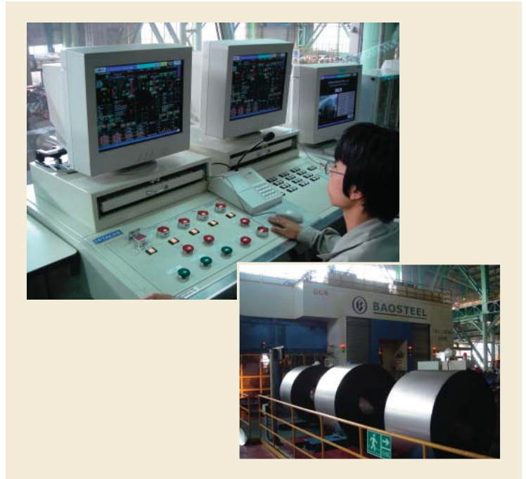
One-person operation in the main control room (above), the mill equipment and cold-rolled coils (below)
