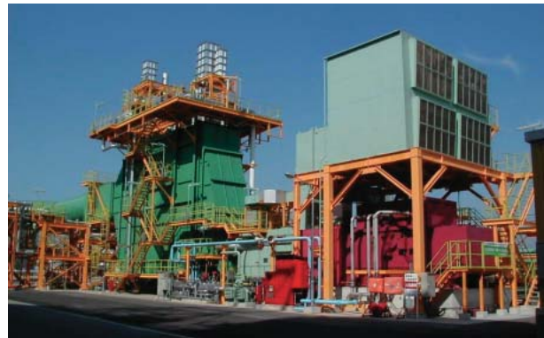
H-25 gas-turbine generator units delivered to Marifu Refinery (left) and Osaka Refinery (right) of Nippon Petroleum Refining Company, LTD.
