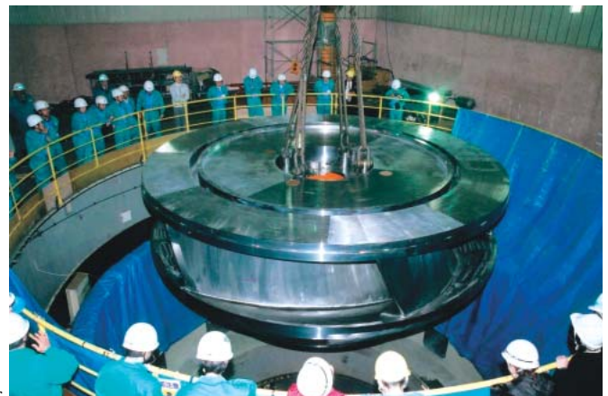
Installation of water-turbine runner
