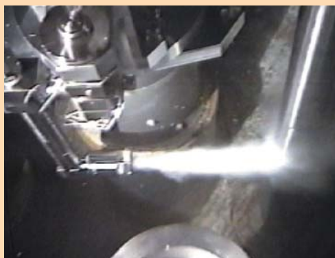
Water jet peening to the reactor internal
