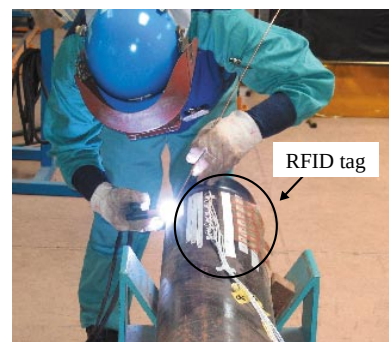
Fig. 2—Scene of Experiment on RFID Tags for Withstanding Welding Heat. By attaching an RFID tag and thermocouple to the piping, the influence of welding heat on the RFID tags was confirmed.
