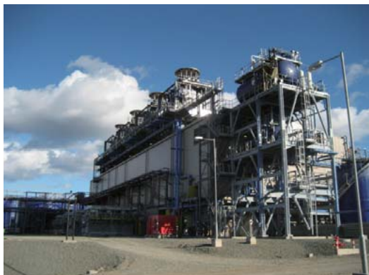
General view of the gas turbine generator building (left) and gas turbine generator building (foreground: lube oil cooler, roof: waste heat recovery unit) (right)
