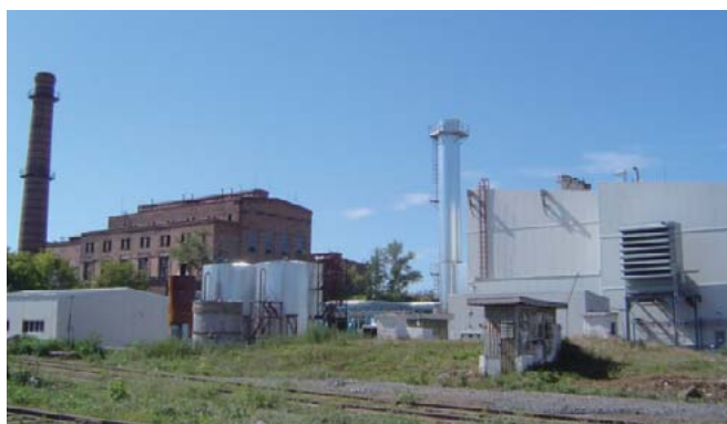
Existing main facility (brown building on left) of the thermal power plant and the H-25 cogeneration facility (white building on right)
