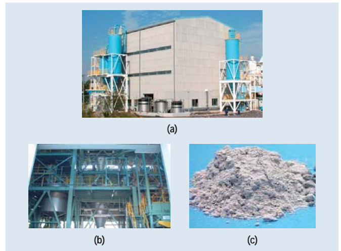
Appearance of artificial zeolitization plant delivered to Hekinan Thermal Power Plant of Chubu Electric Power Co., Inc. (a), inside the building (b), and powdered zeolite (c)
