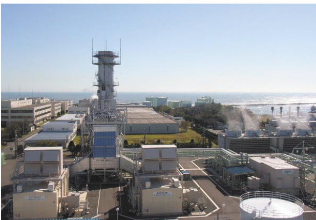
Fig. 1—A View of the Hitachi Rinkai Power Station Unit-2. This unit is a multi-shaft combined cycle power plant composed of two H-25 gas turbines, one heat recovery steam generator, and one steam turbine.
