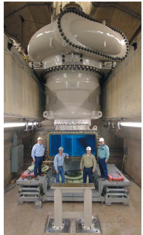
Completion of pump assembly
