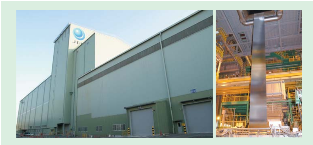
Outside view of West Japan Works of JFE Steel Corporation (left) and galvanizing equipment department (right)
