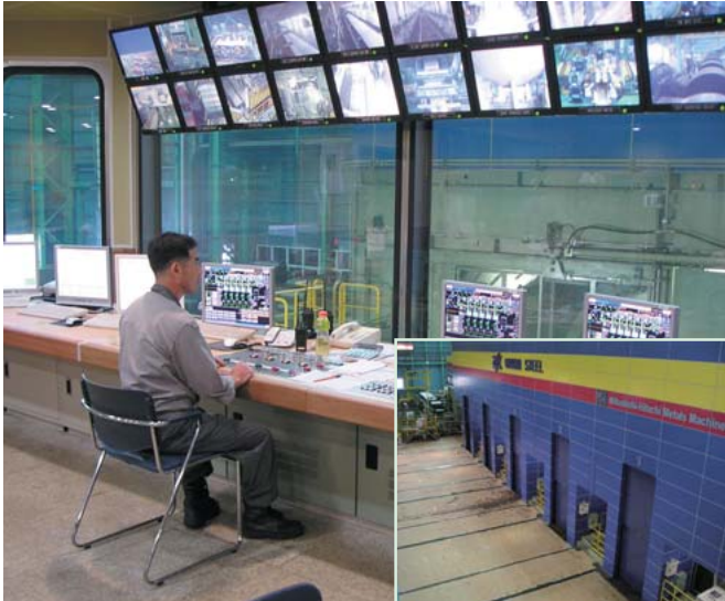
Operation room during one-person operation and cold rolling equipment (right bottom)
