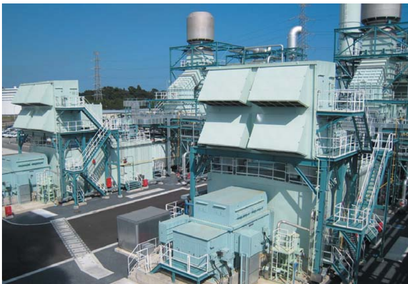
100-MW class high-efficiency H-25 gas turbine combined cycle power generation plants at Nippon Petroleum Refining Co., Ltd.'s Sendai Refinery
