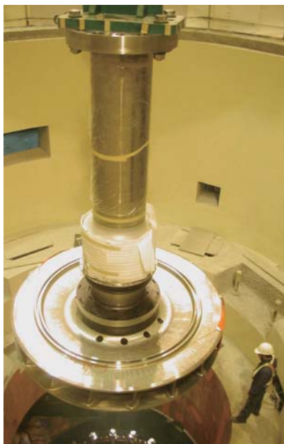
Installation of runner and shaft assembly of the No. 1 55.3-MW hydraulic turbine at Kukuan Power Plant, Taiwan Power Company
