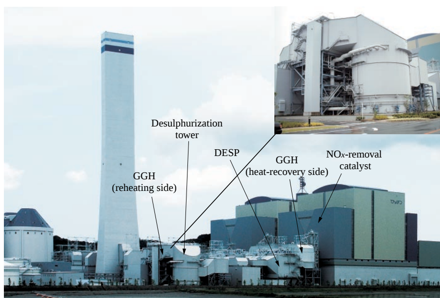
Fig. 1—External View of New Flue-gas Treatment System Applied at Tachibanawan Power Station Unit 2 of Electric Power Development Co., Ltd. At Babcock-Hitachi K.K., we are contributing to environmental protection all over the world through development and practical application of new flue-gas treatment systems for efficiently cleaning up flue gas from thermal-power-plant boilers.
