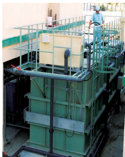
Fig. 9—MBR Facility for Construction-worker Camps. The appearance of an MBR facility installed at a construction-worker camp in Dubai City in 2007. The facility has a treatment capacity of 250 m 3 /d in processing human wastewater for about 1,500 people.
