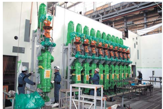
Fig. 5—HCU Module Assembly (2). HCUs were installed and anchor bolts were embedded on SC walls (March 2007).
