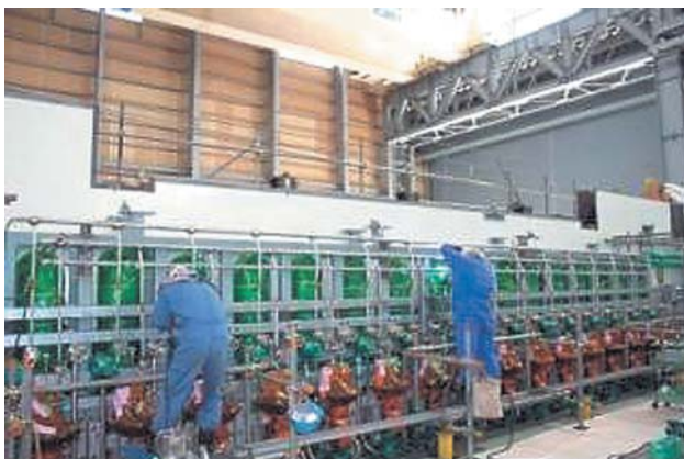
Fig. 6—HCU Module Assembly (3); Process Piping Welding. Process piping was welded and installed after HCU installation. This room module was shipped after all piping in the room was installed (May 2005).
