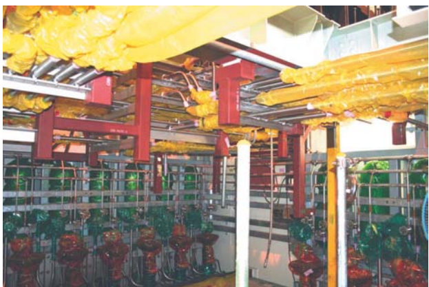
Fig. 7—HCU Module Assembly (4); Process Piping Installation. Installation of piping and support for the piping was completed (October 2007).
