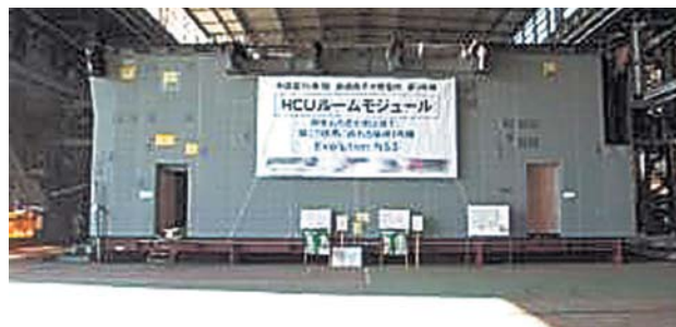
Fig. 8—HCU Module Assembly (5). Panoramic view of HCU room module is shown. This is the final phase before shipping (January 2008).
