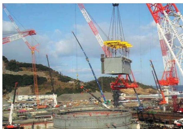
Fig. 9—HCU Module Installation. HCU was carried in by crawler crane at Shimane-3 site (February 2008).
