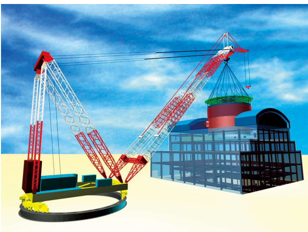
Fig. 5—Image of RCCV Lower Liner being Lowered into Position in Steel Frame. The image shows the lower liner being lowered into the steel frame which has already been constructed and from which the temporary roof has been removed.
