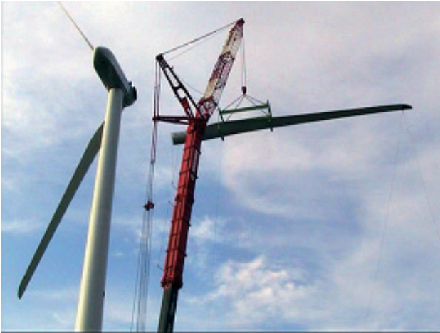
Fig. 6—Blade Being Attached to Hub at Top of Tower. Assembling the rotor in the air one blade at a time saves on ground space.
