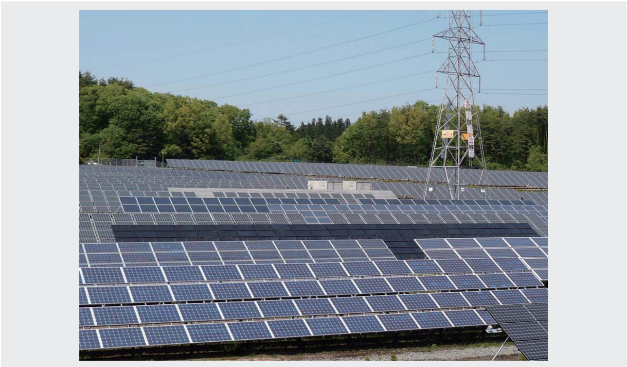
Fig. 1—Hokuto Site for Verification of Grid Stabilization with Large-scale Photovoltaic Power Generation Systems Operated by New Energy and Industrial Technology Development Organization (NEDO). View of megasolar generation panels at a solar power generation system of approximately 2 MW under construction at Hokuto in Yamanashi Prefecture is shown.
