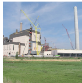
Coal-fired power plants (under construction)
