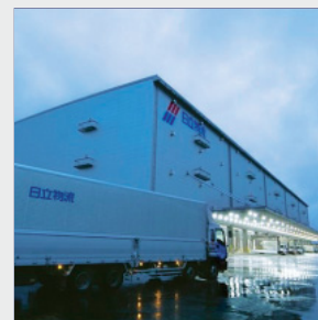
Hitachi Transport System has opened a joint distribution center for the toilet-ries industry —East Japan PFC (Platform Center)—
