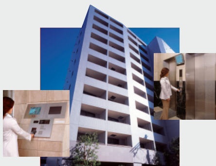
IT condominium systems
