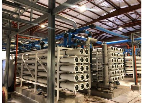
The seawater desalination and water reuse integrated system (Reverse Osmosis (RO) membrane)
