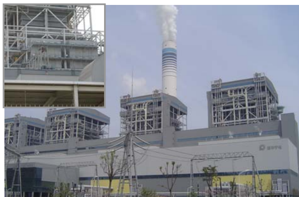
Fig. 2.1 Flue Gas Denitration Equipment of Ninghai Power Plant, China (enlarged photo at top left)
