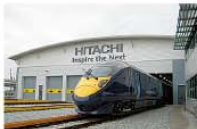
Ashford Train Maintenance Centre
