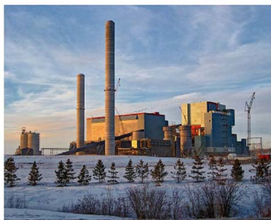
Fig. 2.2 The first supercritical coal fired power plant in North America
