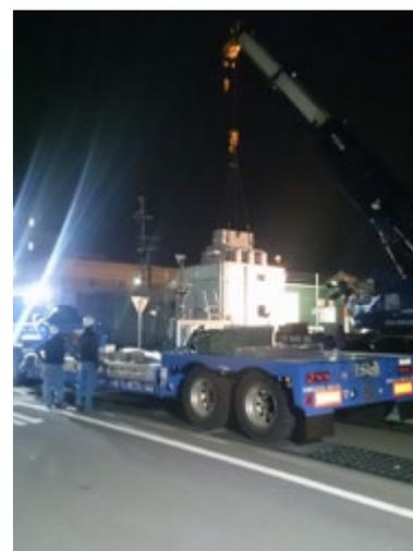
Disposing of waste materials (large transformers) containing PCBs.
