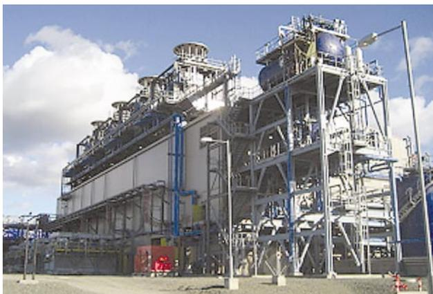
*Fig. 5—H-25 Gas Turbines in Sakhalin II Project in Russia. Hitachi delivered four H-25 gas turbine generation equipment units to the Sakhalin Energy Investment Co., Ltd., for use in a land-side plant that processes gas and oil extracted from the seabed off the eastern shore of Sakhalin Island in Russia.*
