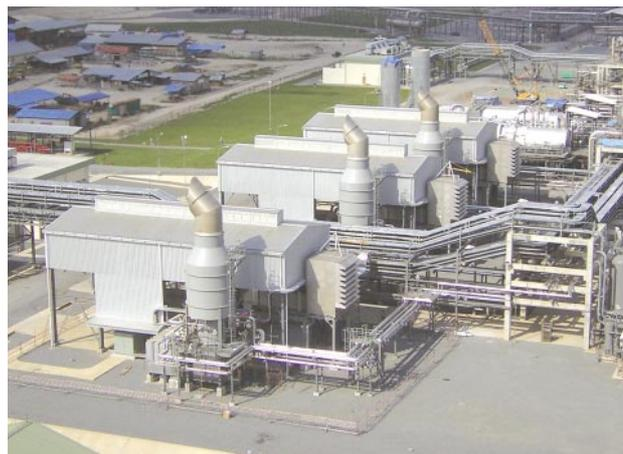
*Fig. 7—Overview of Betara H-25 Plant. Hitachi delivered three H-25 gas turbine generator sets to Betara plant in Indonesia.*
