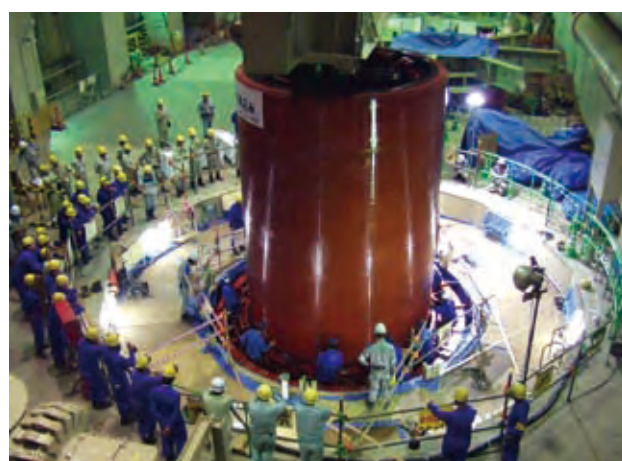
Fig. 2—Assembly of Motor-generator for Omarugawa Power Plant of Kyushu Electric Power Co., Inc.
