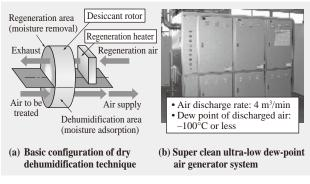
Fig. 10—Principles of Super Clean Ultra-low Dew-point Air Generator Technology and Equipment Photograph. The system works on the principle of dry dehumidification and consists of three desiccant rotors connected in series.
