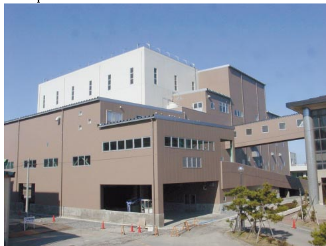
System delivered to Itoigawa Area Broader Administrative Association Scale: 70 t/d (35 t/d × two furnaces)
