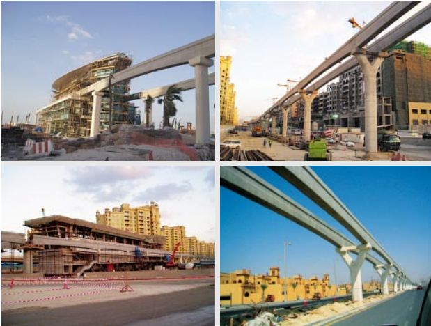
Fig. 6—Civil and Structural Work now in Progress. Some of Hitachi's manufactured systems and equipment have already been delivered and are now beginning to be installed.
